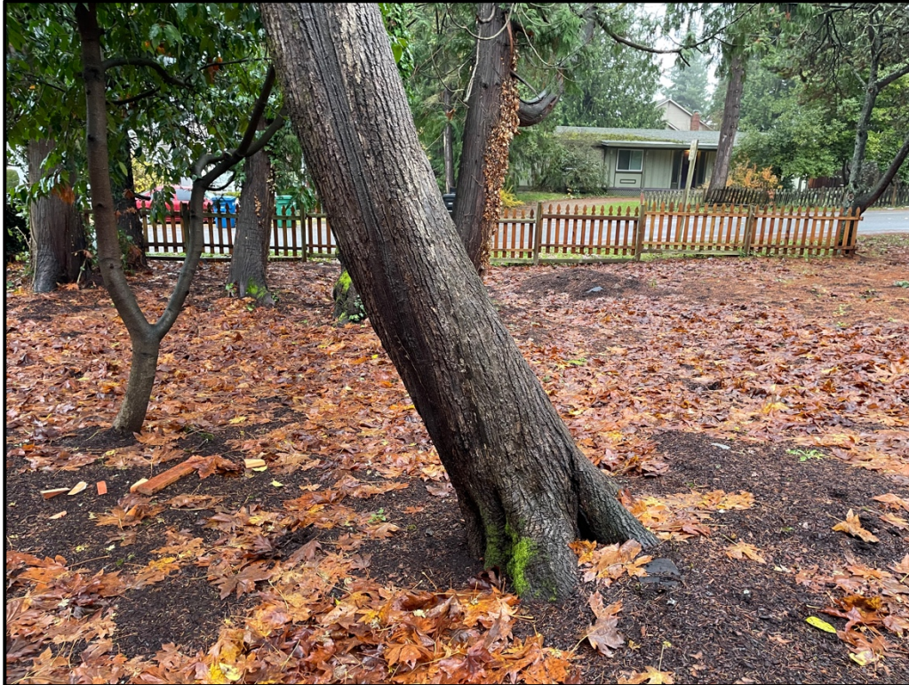
Photograph 2. The base of tree 94. This tree poses a hazard to the house north of the property and should be prioritized for removal.
